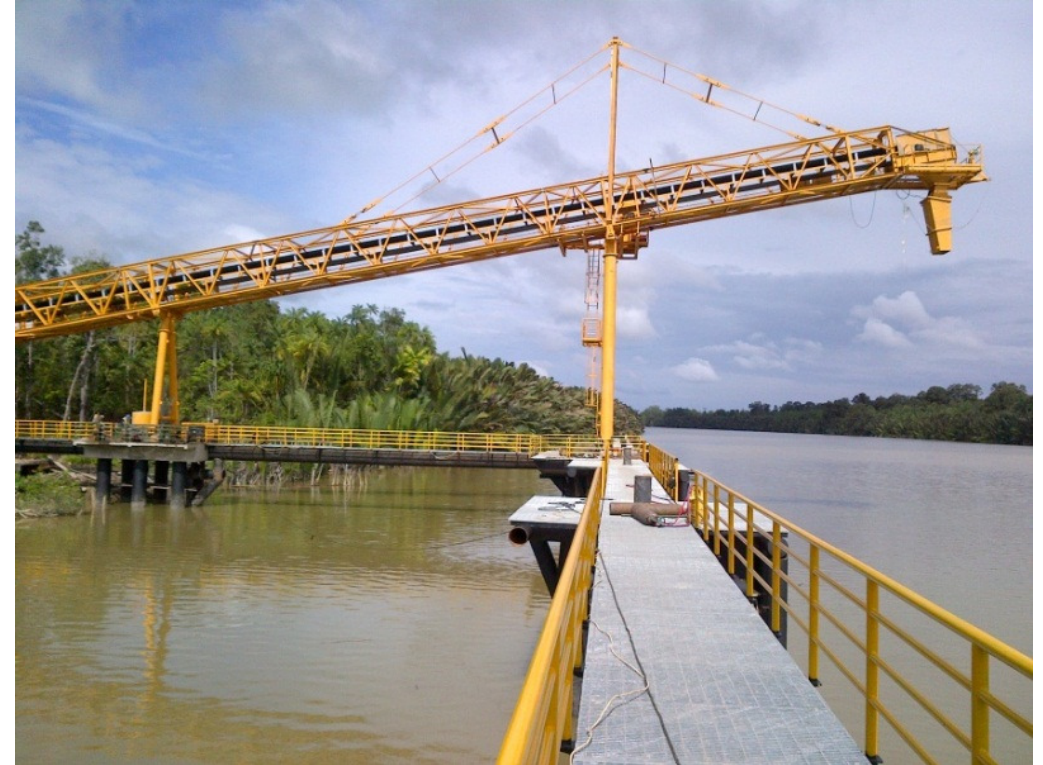
Construction of Jetty, East Kalimantan
