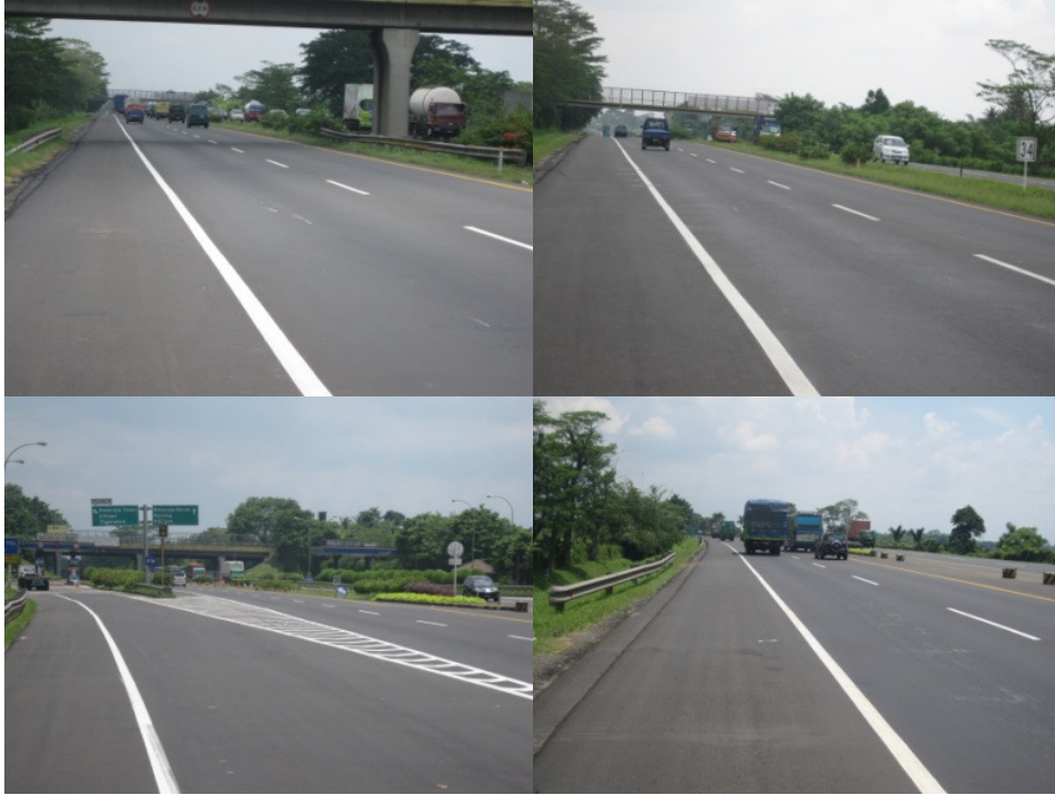
Improvement on Tangerang-Merak Toll Road
