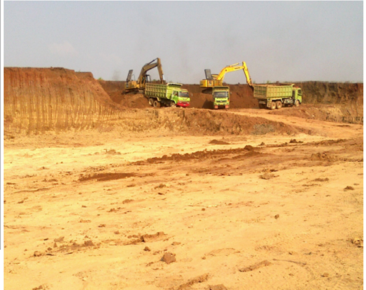
Cut and Fill Work in Phase 3
